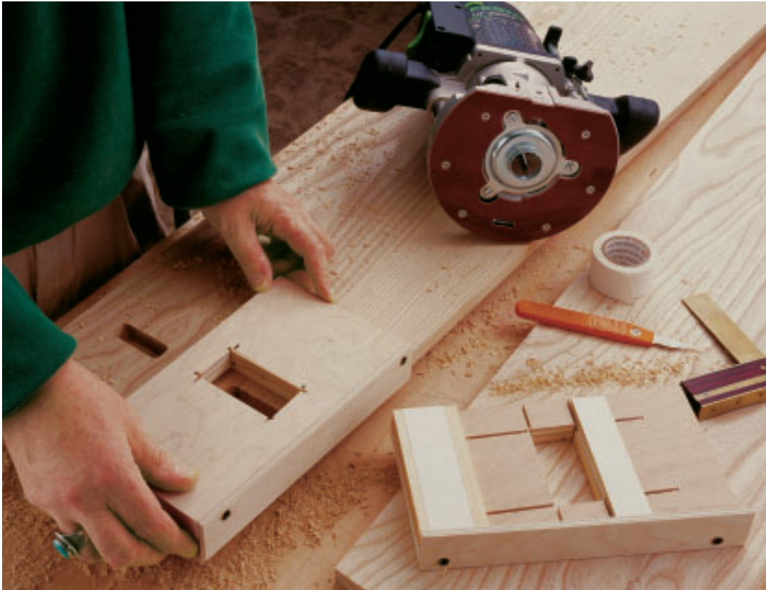
Photo C: To cut the through mortises in the sides, you need a left-handed and a right-handed router jig.
